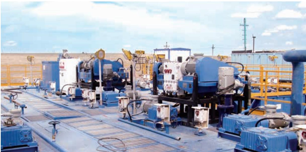
KOSUN decanter centrifuge can meet with different requirements of mud treatment under various drilling conditions, which separates particles over 2 $\mu$ m. After treatment, the mud can achieve ideal viscosity and proportion, results in better recycling, high efficiency, material saving and environment protection.
